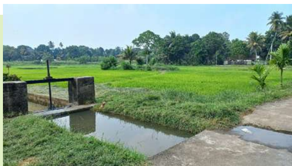
Figure 4. Sri Lankan traditional water management and control system used to fulfill water needs for paddy cultivation. © Olupathage Tharanga Dilhari Silva
