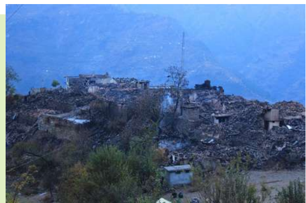
Figure 9. Kotla village after the fire in November 2015 that gutted the entire village © Madhusudan Singh
