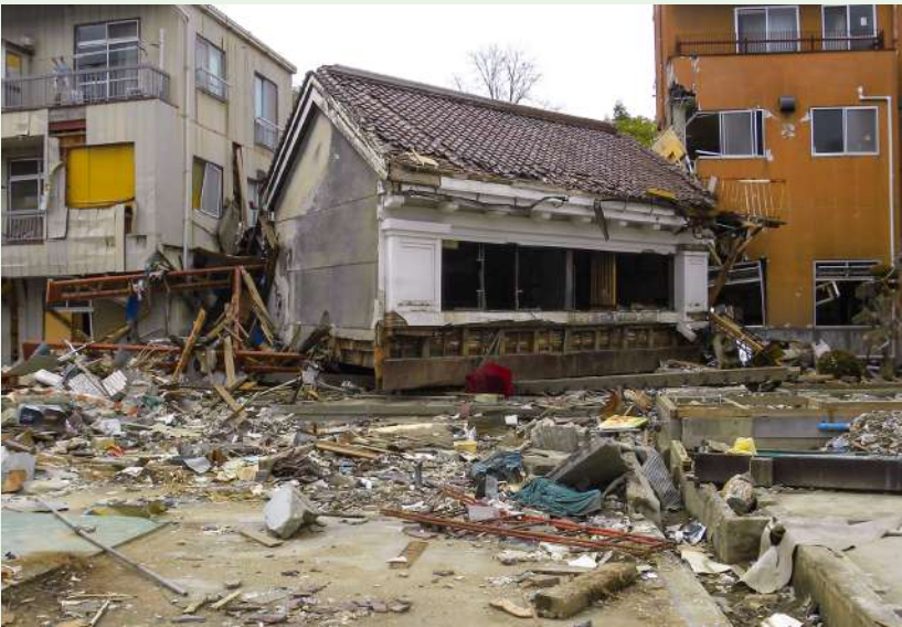
Building collapse caused by tsunami in eastern Japan, 2011. Photo: Board of Miyagi prefecture.
