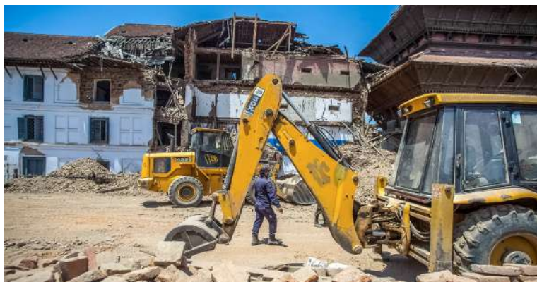
In the immediate aftermath of the earthquake, clearing operations underway in Kathmandu, Nepal, 2015. Photo: Tapash Paul/Drik.
