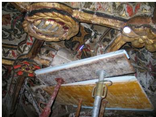
Protective and isolating layer between the wall painting and shoring in the church of Freixo de Espada à Cinta, Portugal, 2007. Photo: Esmeralda Paupério.
