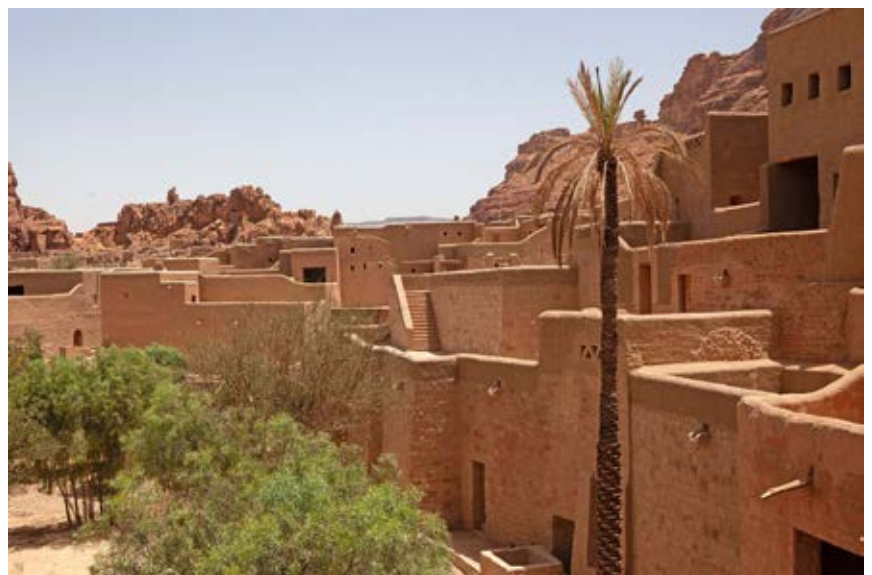
▼ Restored mud houses in AlUla Old Town.
