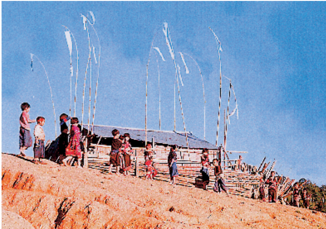
Plate 1. A Lahu Nyi village temple: structurally unique and set apart from other village buildings
