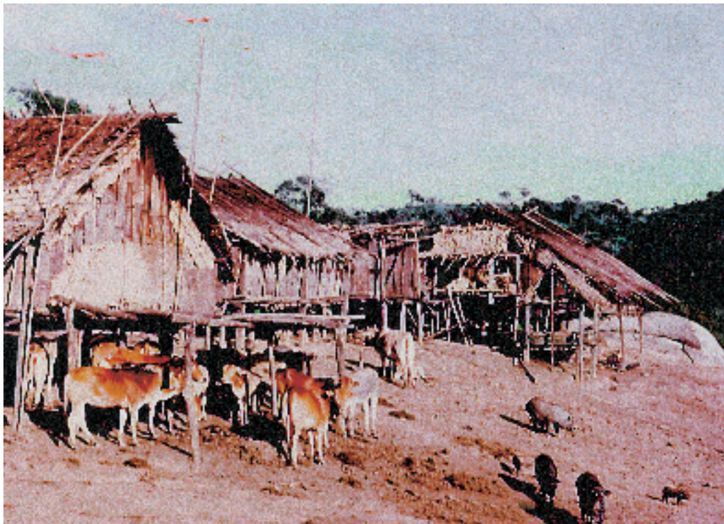
Plate 2. Bamboo and wood houses with grass- or leaf-thatched roofs and set on piles: Typical Lahu Nyi domestic architecture in upland North Thailand in the 1960s
