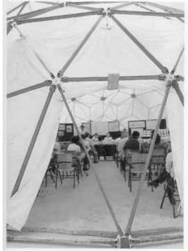
Figure 5. Demountable geodesic dome prototype, devised by A few years later, I arranged for R. Buckminster Fuller and Shoji Sadao in 1981, for covering
