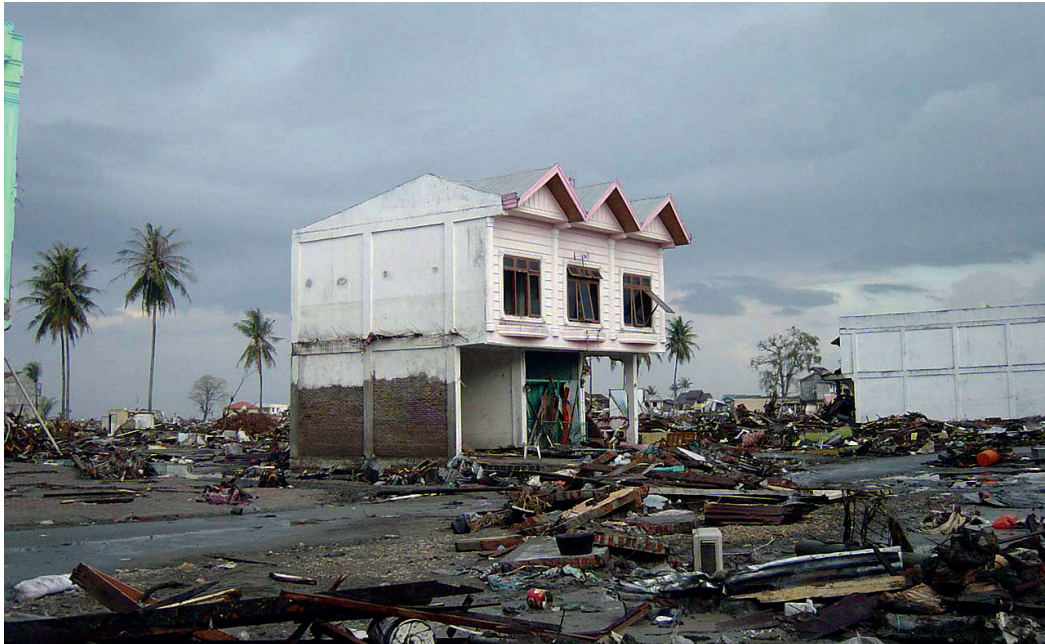
Figure 2. Impact of tsunami of 26 December 2004 at Banda Aceh (photo Michael L. Bak at Wikicommons)
