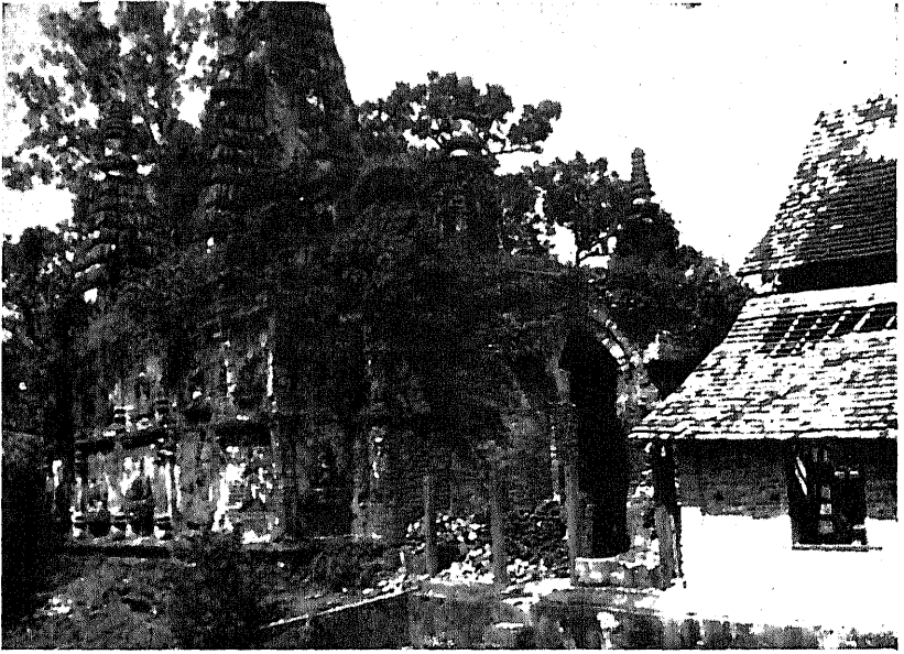
The Seven Spires E. Façade
