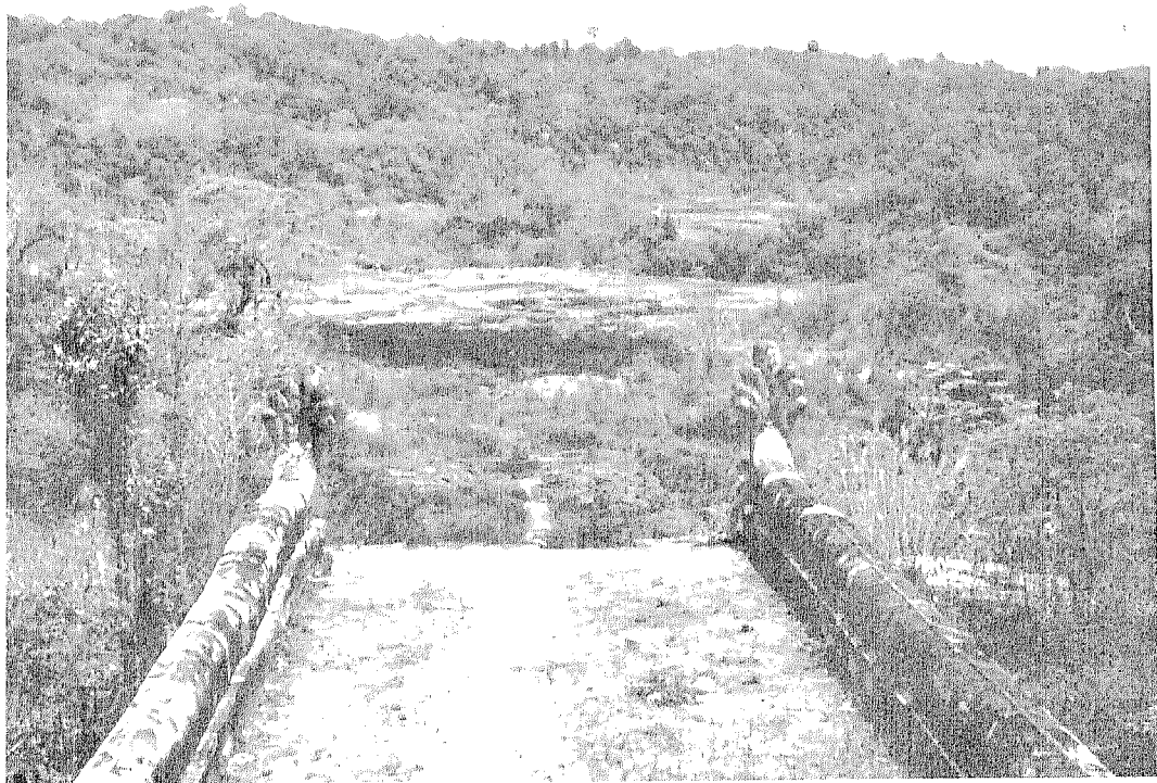
Naga Balustrades at Top of Grand Stairway, Looking North
