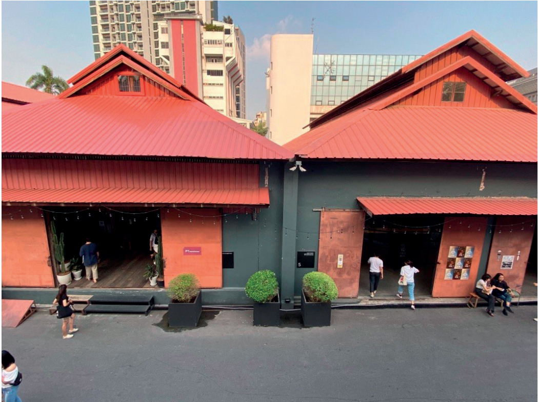
Figure 13. Warehouse 30 today (photo: Warehouse30.com)
