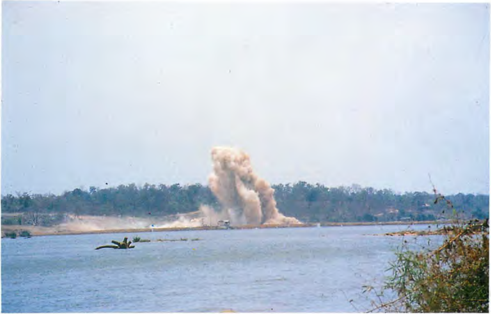
Figure 10. One of the thousands of detonations used in removing the rapids and excavating the streambed for Pak Mun Dam.
