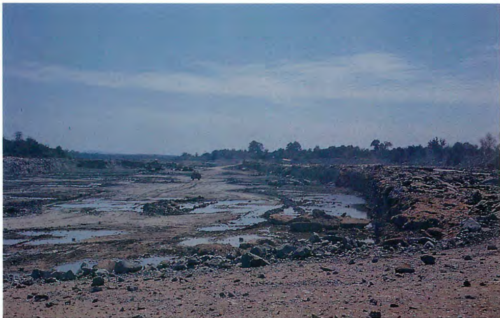
Figure 12. Completed excavation, with water held back by coffer dams.
