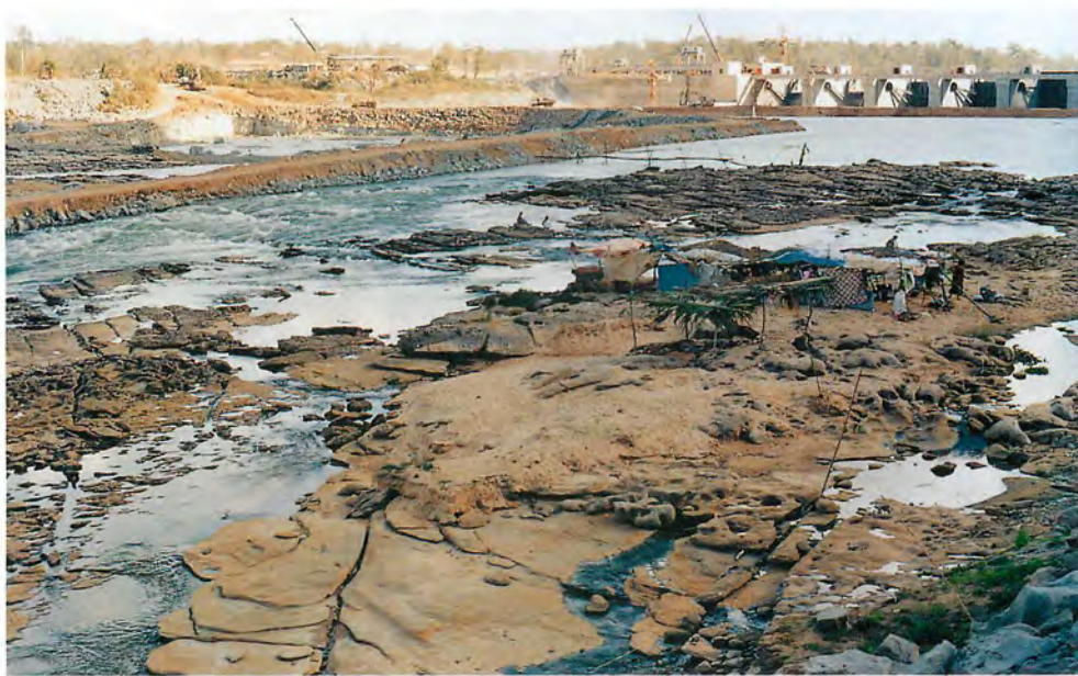
Figure 9. Pak Mun Dam, with five of its eight turbines. Fish ladder not yet installed. Immediately downstream is a coffer dam within which blasting and excavation was going on (December 1993).
