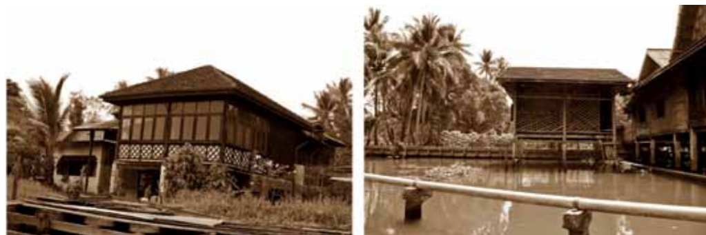
Figure 3. Wooden houses with hip roof and simple gable roof
