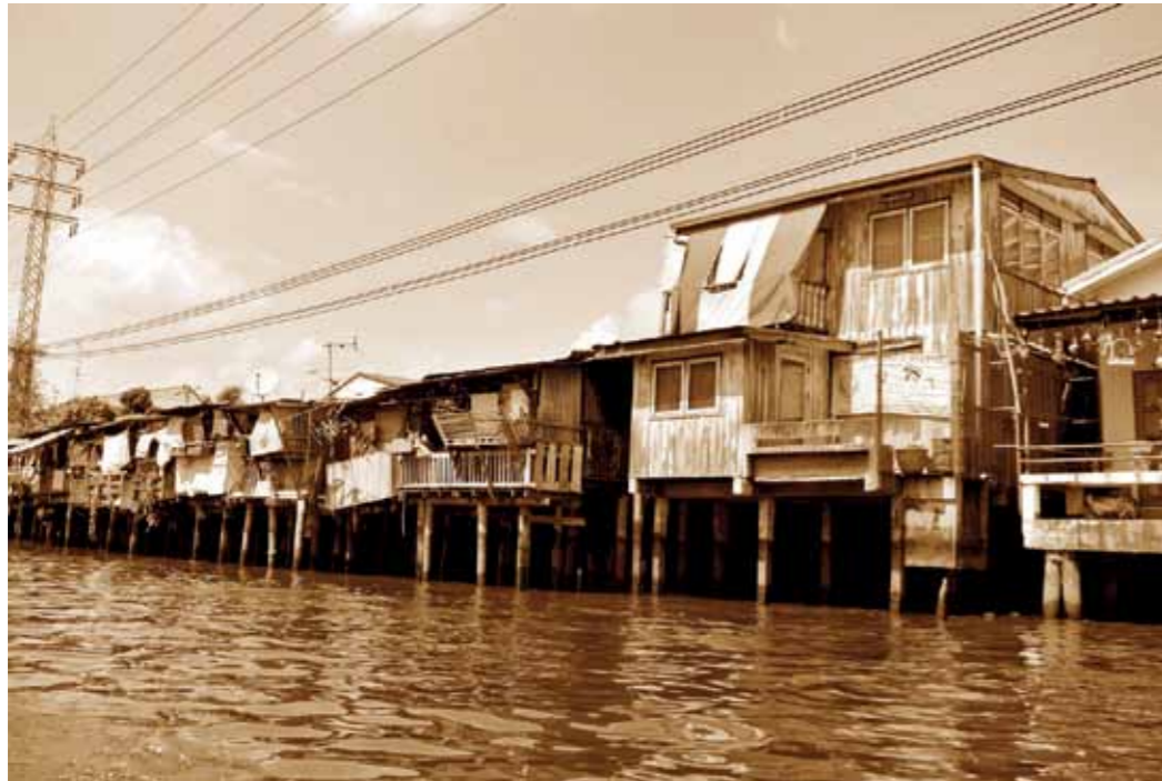
Figure 2. Wooden houses along Khlong Bang Luang
