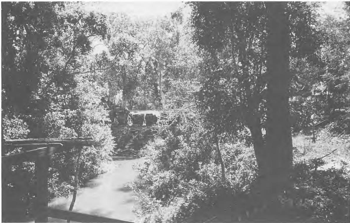
Fig. 2 The present Siem Reap canal has scoured a channel four feet below the original canal bottom shown by the remains of the bridge footings in the center of the photograph. The terrace on the right shows the original canal bottom.
