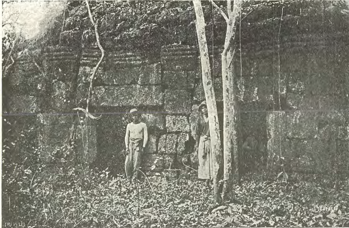
Cloisters along the North Wall; view from inside the walls.
