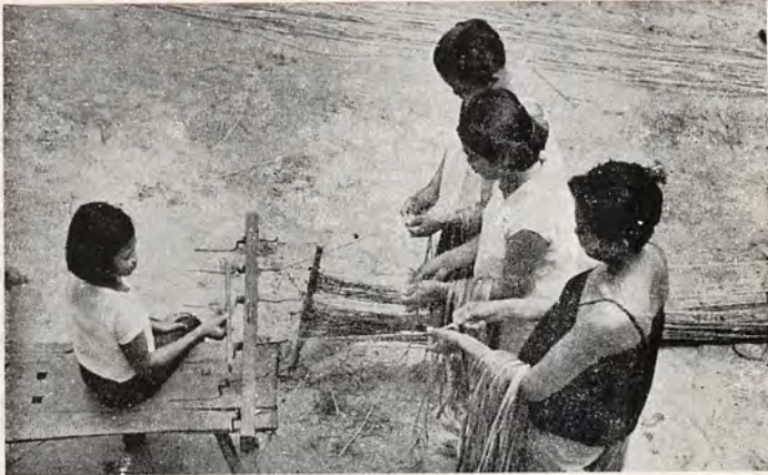
Fig. 5. Twisting the dry strips of jute bark into cords.
