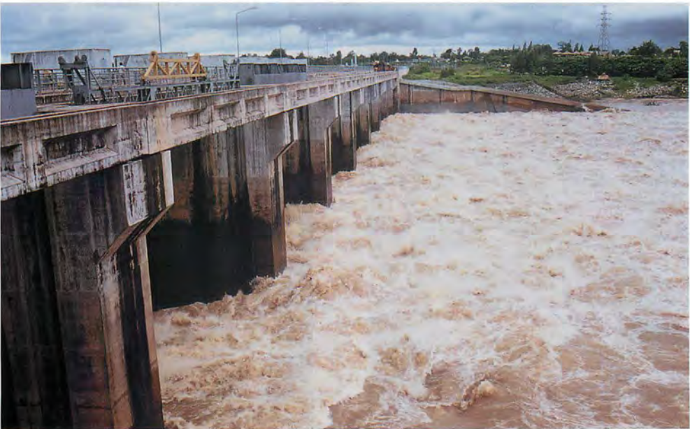
Figure 7. Pak Mun Dam with spillways wide open. The violently turbulent conditions continue down the reservoir outflow to the Mekong mainstream; date unrecorded. Few if any of the naturally occurring fish species of the Mun River can survive such conditions. Such flooding is one of the reasons it is objectionable to call Pak Mun Dam a “run-of-the-river” installation; (courtesy of The Nation ). See Fig. 15.
