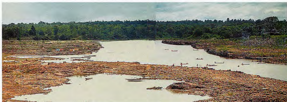
Figure 4. Partially exposed bed of Mun River (held back by coffer dam) immediately downstream from Pak Mun Dam. Note the relatively deep channel (with fishing boats) on right side of river. This is the main pathway taken by migratory fish moving up the Mun River. Also note extensive hard-rock reef on the left side blocking the way to the fish ladder. EGAT excavated a narrow channel about 1–2 m deep through the reef as access for fish to the fish ladder (see also Fig. 5) (courtesy of Sanay Pholprasith).
