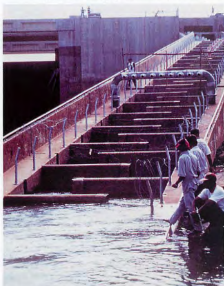
Figure 9. Completed fish ladder ready for fish, viewed from reservoir outflow with water conditions favorable to fish movement upstream (courtesy of Prapard Phanaram and EGAT).
