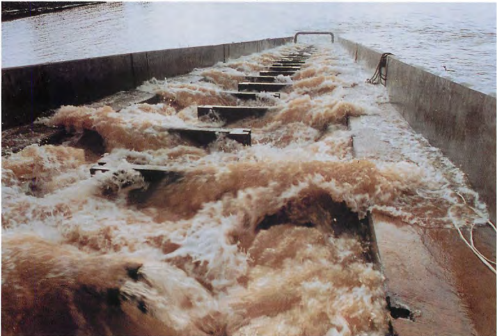
Figure 12. Close-up of fish ladder looking down from the dam. Current in reservoir outflow favorable but current in fish ladder far too strong; 15 June 1994 (courtesy of Prapard Phanaram and EGAT).
