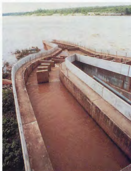
Figure 10. Fish ladder from above looking down. Flow in reservoir outflow too strong and flow in fish ladder too weak; date unrecorded (courtesy of The Nation ).
