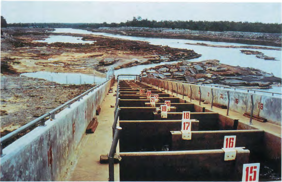
Figure 6. Fish ladder during late stage of construction viewed from top of dam before completion of construction. Note narrow artificial channel through reef leading to mouth of fish ladder (courtesy Prapard Phanaram and EGAT). Compare with Fig. 4).
