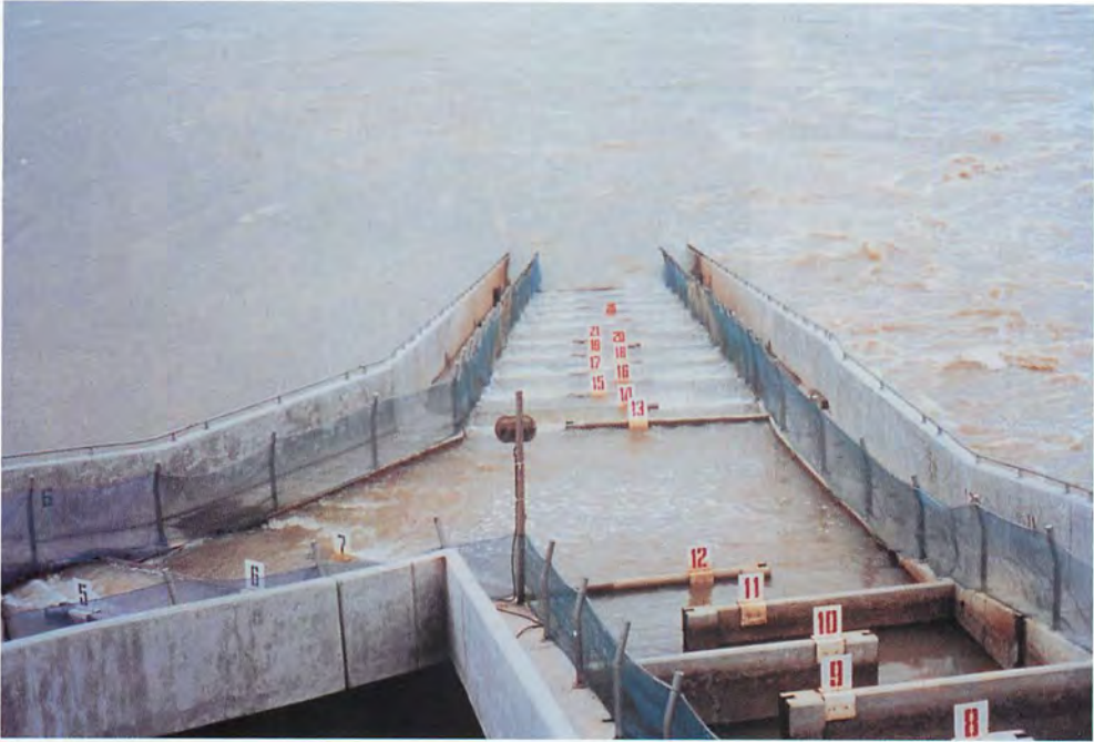
Figure 11. Close up of fish ladder looking down from dam. Water flow in reservoir outflow and in fish ladder favorable for fish; date unrecorded (courtesy of Sanay Pholprasith).
