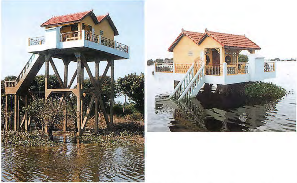
Figures 2,3. Two views of an elevated structure (ca. 10 m high) in Prek Toal Village illustrating the dramatic seasonal variation in water levels of Tonle Sap. Structure in late February when water levels are declining (left). Same structure in September as water levels approach annual maximum (right).
